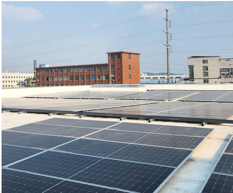
V-NP-F Flat Installation — Vandewiele TPO project
