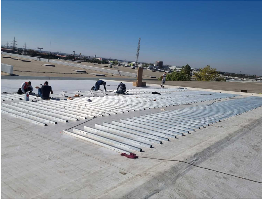
V-NP-FP Flexible Panel Bracket — purpose-built for lightweight modules
