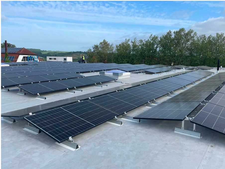
V-NP-EW East-West Installation — butterfly configuration on TPO roof
