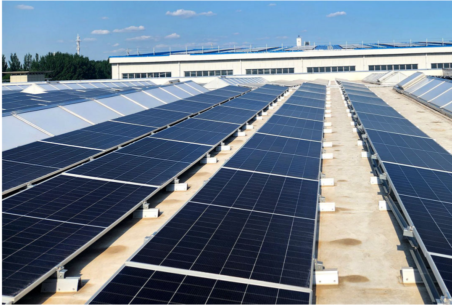
V-NP-S South-Facing Tilted Installation — Boysen TPO project
